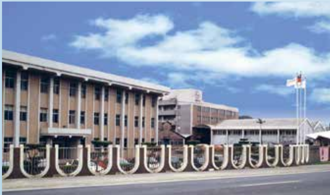
三峽廠 San Hsia Plant
