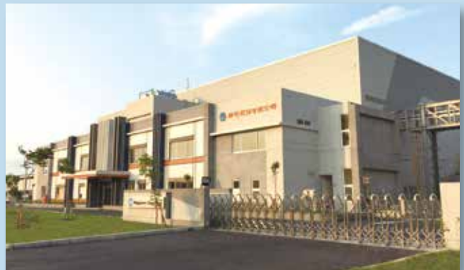
屏東廠 Ping Tung Plant
